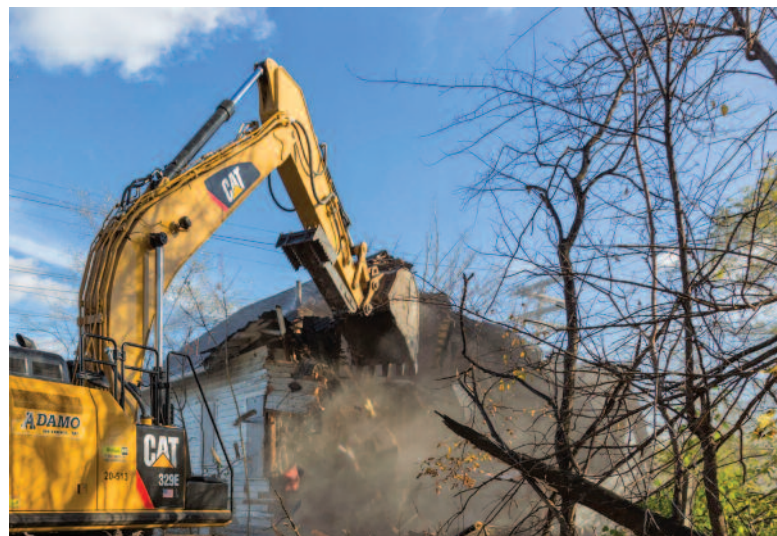
▼ Detroit residential blight removal is underway.
